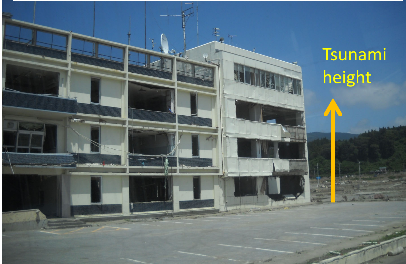
Rikuzentakata city office
